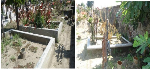
Figure 9 Graves with concrete curb
